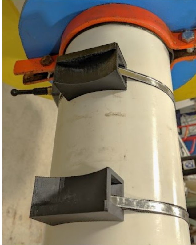
Figure 4.8: Mounting brackets for flow meter housing installed onto spar buoy.
