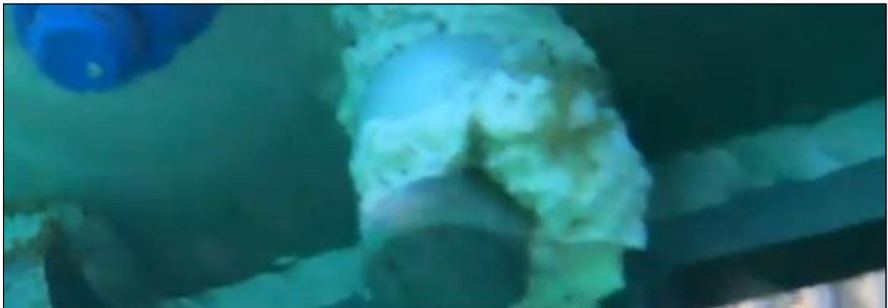
Figure 28: Corroded fairlead anode.
