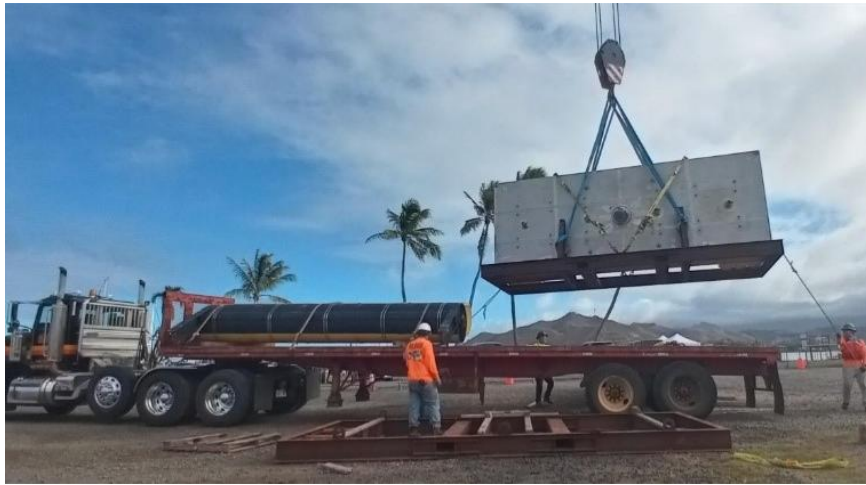
Figure 39 - SeaRAY and heave plate loaded onto truck.
