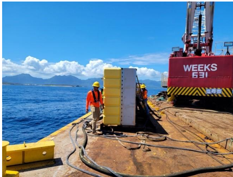
Figure 27 - Final connection of heave plate to SeaRAY with bridle lines and mooring.
