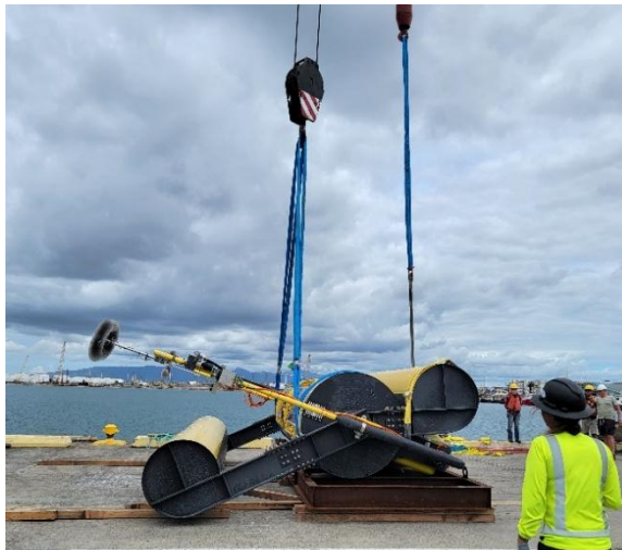
Figure 18 - WPS with crane attachments.
