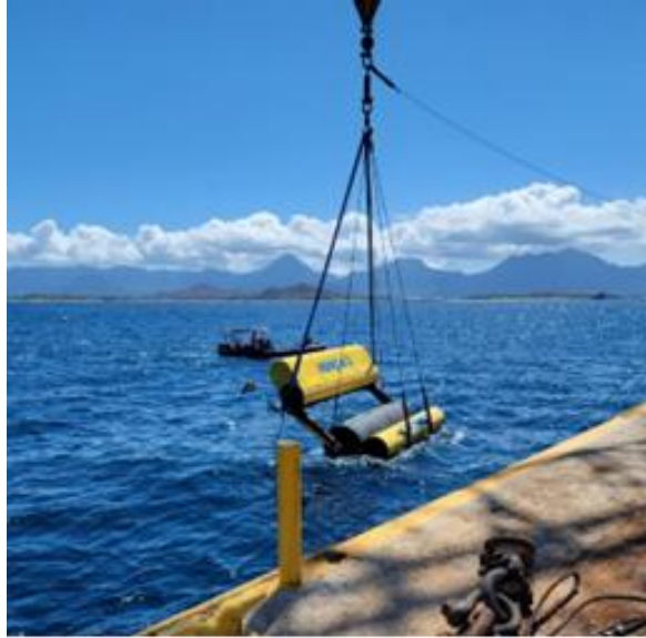
Figure 28 – SeaRAY placed into the water via crane.
