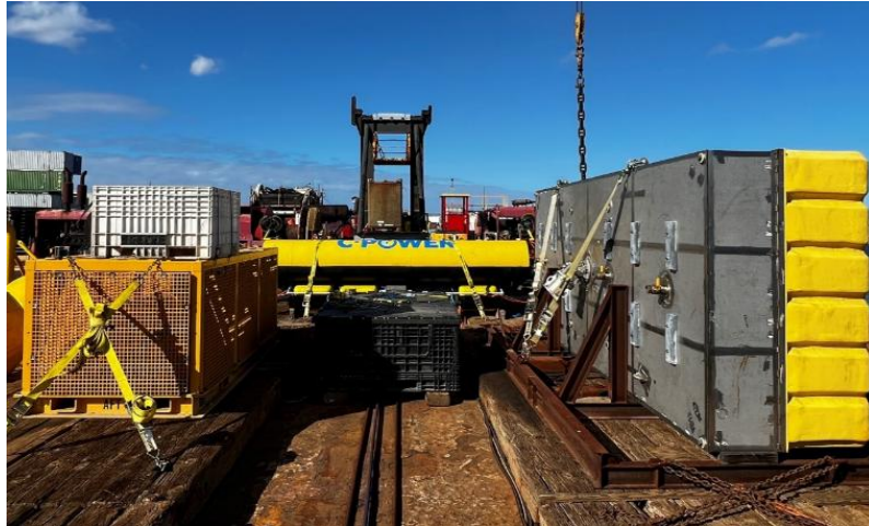
Figure 24 - SBU (left) and heave plate (right) loaded onto barge.
