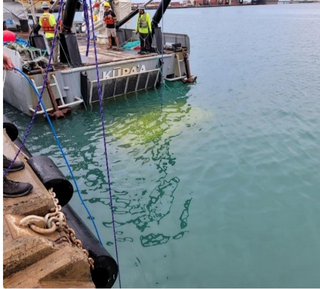
Figure 23 - SBU lowered into water.
