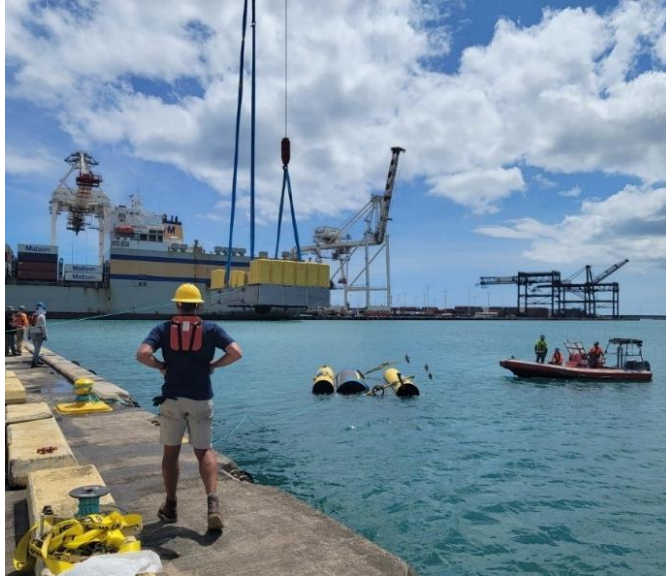
Figure 19 - Heave plate maneuvered into position while RHIB tends to WPS.
